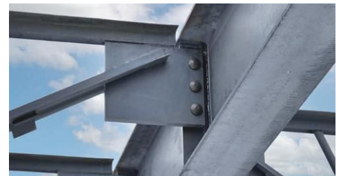
Joist reaction point occurs at beam centerline
