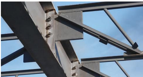
Flush-frame connection designed for efficiency
