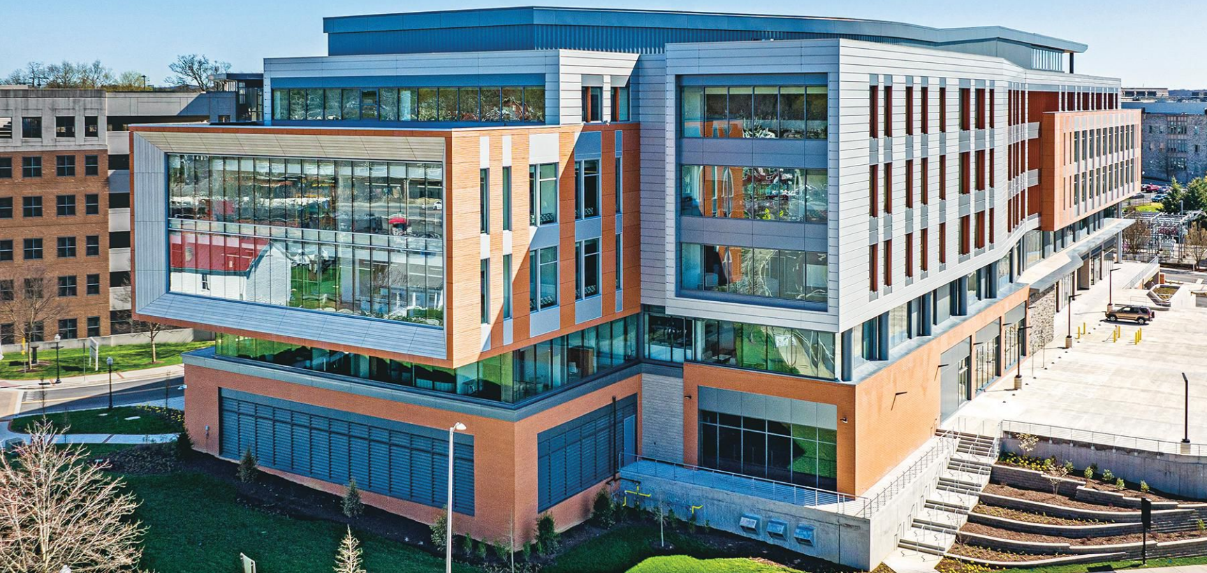
Gilbert Place at Virginia Tech Blacksburg, Virginia — QuadCore® KarrierPanel®, Designwall 4000 and Designwall 2000
