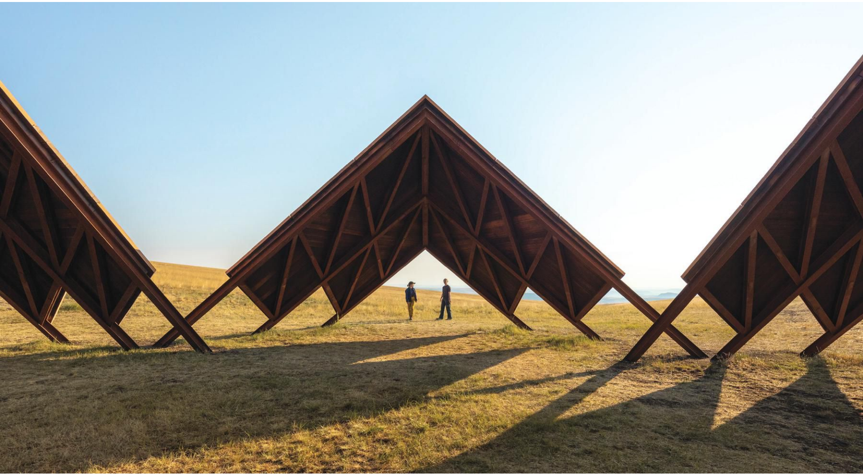
The Geode touches the ground lightly (above), tied to the earth via micropiles. Arlen Hlusko performs at the Geode in August (left).
